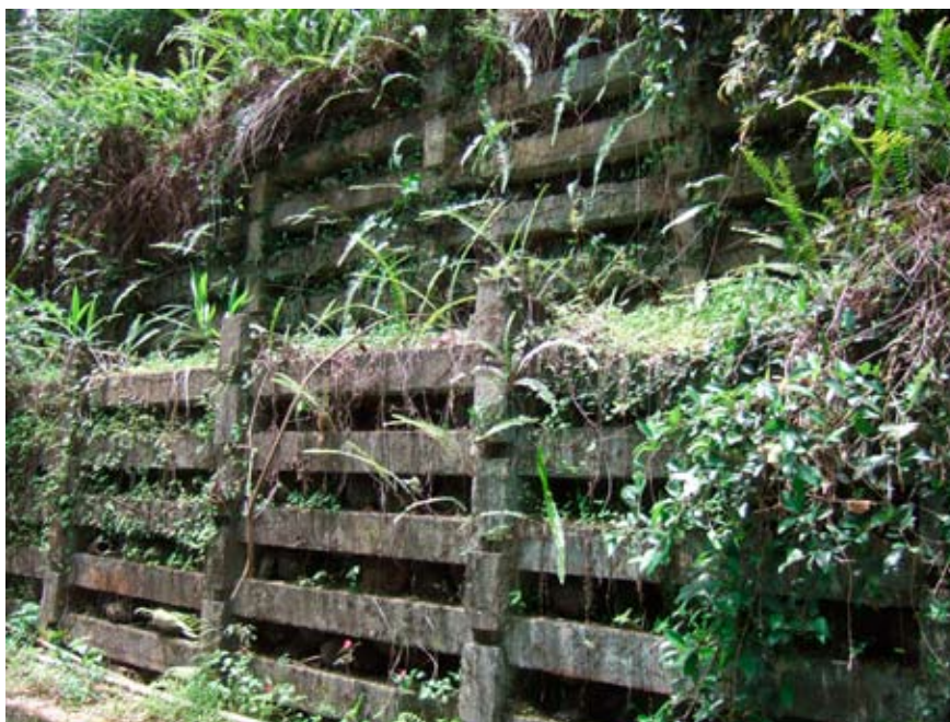
格籠壩式擋土牆 Arch Dam Revetment
