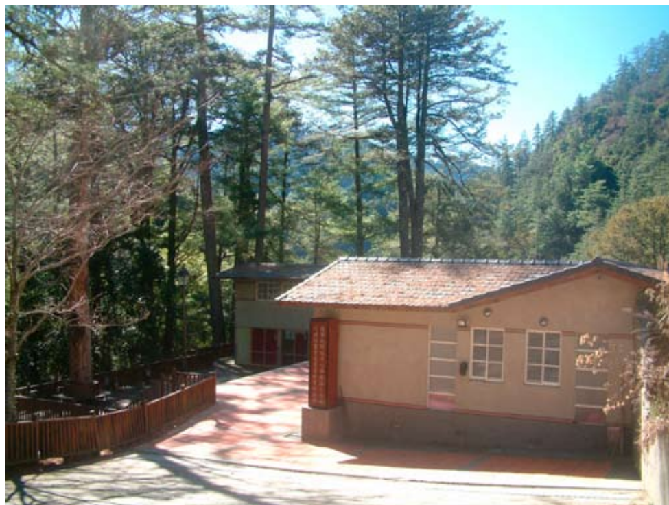
畢祿溪工作站 Piluchi Working Station
