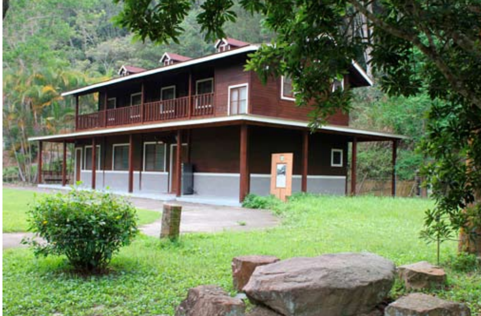
肖楠木屋教室 Wooden Classroom of Taiwan Incense Cedar
