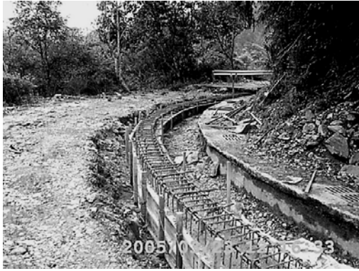
【3】土釘結合地樑完成 【3】Combination of soil nail and Ground beam
