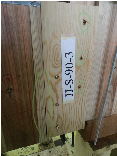
Fig. 5. Self-tapping screw head penetrating through the spline at the connection.
