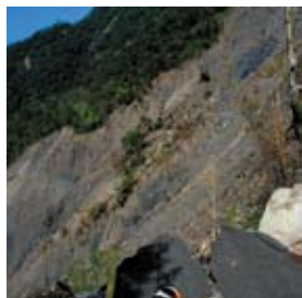
4.9 K~5.4 K嚴重崩塌，長約300 m
